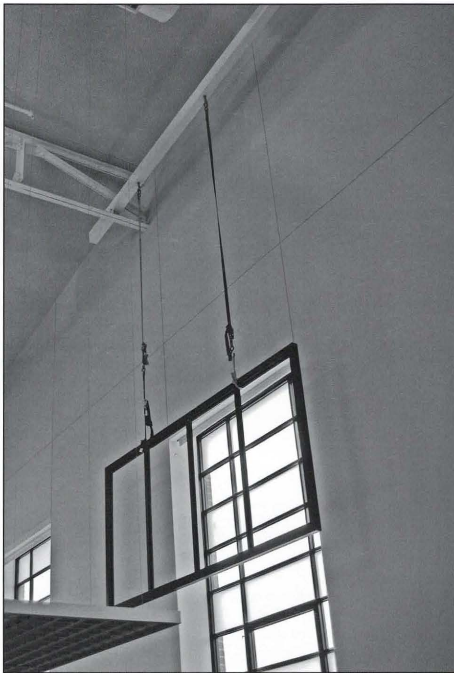
Detail of hanging system before panel placement.
